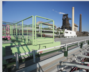
Air cooler with an automatically travelling cleaning platform
