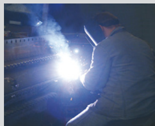
Repair welds on a leaky tube bundle.
