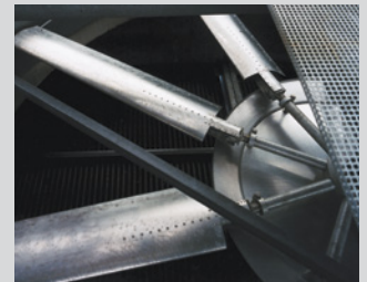
Maintenance work on fans.
